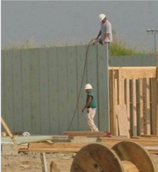
Figure 1.4-A Unprotected Storage of Water-Sensitive Materials
