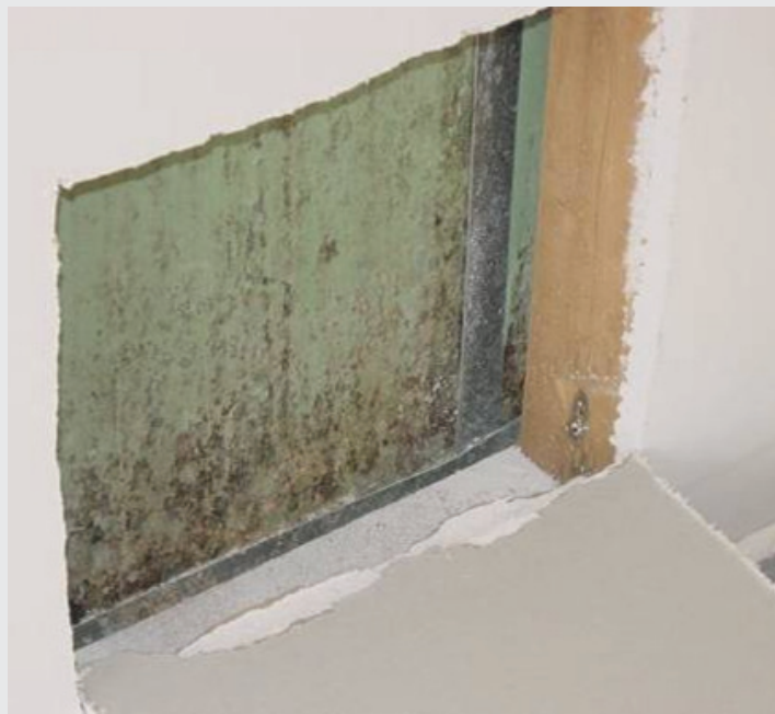
Figure 1.4-C Mold Growth from Wetting of Exposed Water-Sensitive Materials—Example 1
