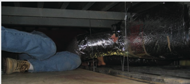
Figure 4.3-C System Location Limits Access
