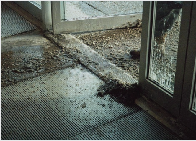
Figure 2.5-A Inadequate Track-Off Design for Local Conditions Photograph courtesy of Hal Levin.
