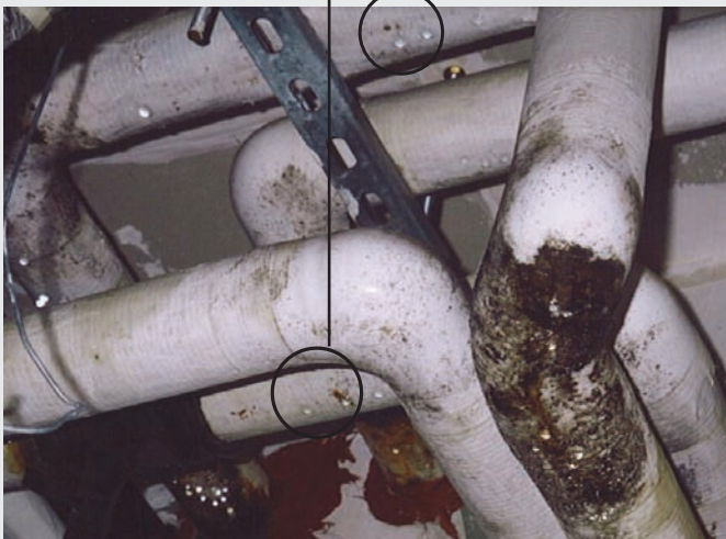
Figure 4.2-A Condensation Drips and Mold on Pipe Insulation
