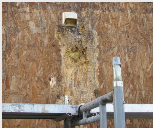
Figure 2.1-C Damage from Failure at Vent Penetration
