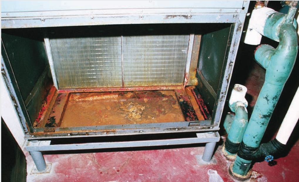
Figure 4.1-A Drain Pan that was Poorly Designed and Maintained
