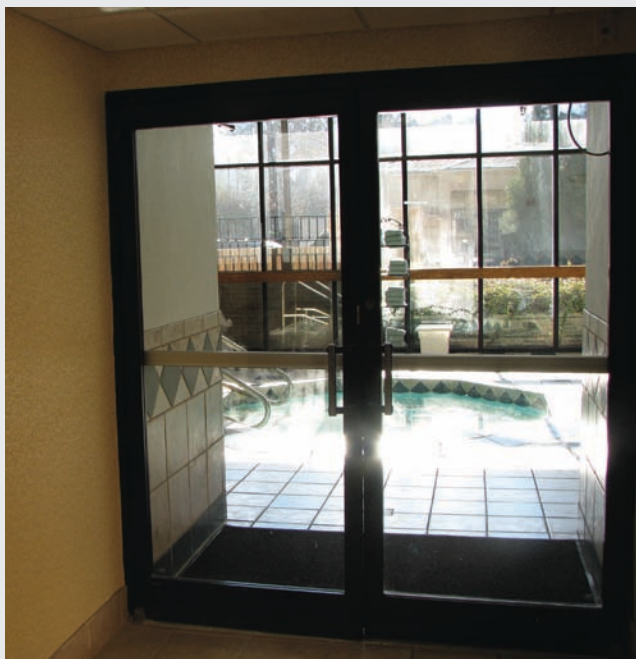
Figure 6.4-B Ill-Fitting Double Glass Doors
