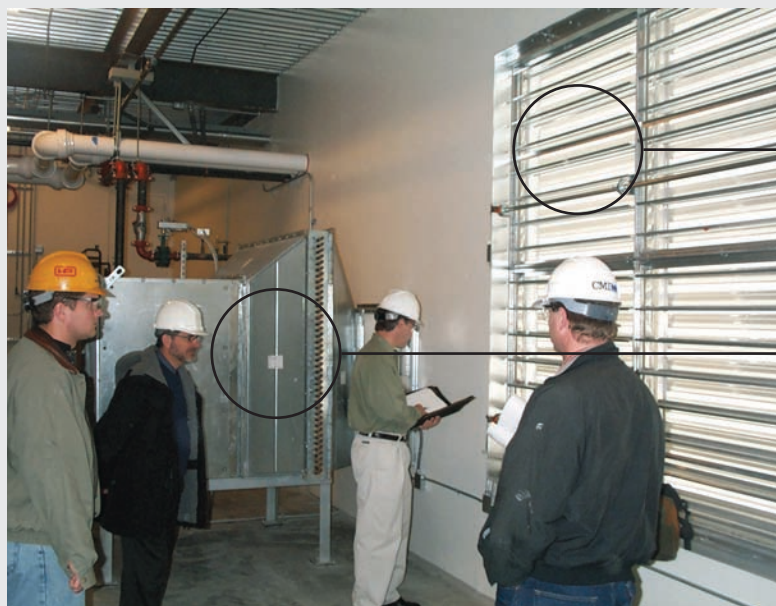
Figure 7.2-A Minimum Outdoor Air Fan and Main Outdoor Air Dampers of a Build-Up HVAC System
