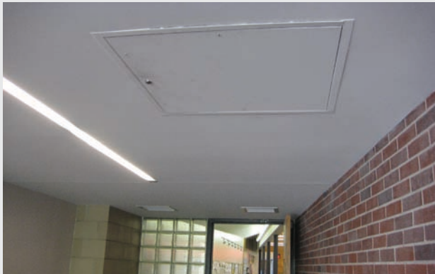
Figure 4.3-A Access Door to Systems
